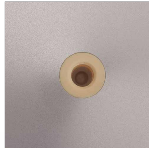
The plastic bushing in the platter forms the counterpart to the platter axis and only has to absorb horizontal forces
